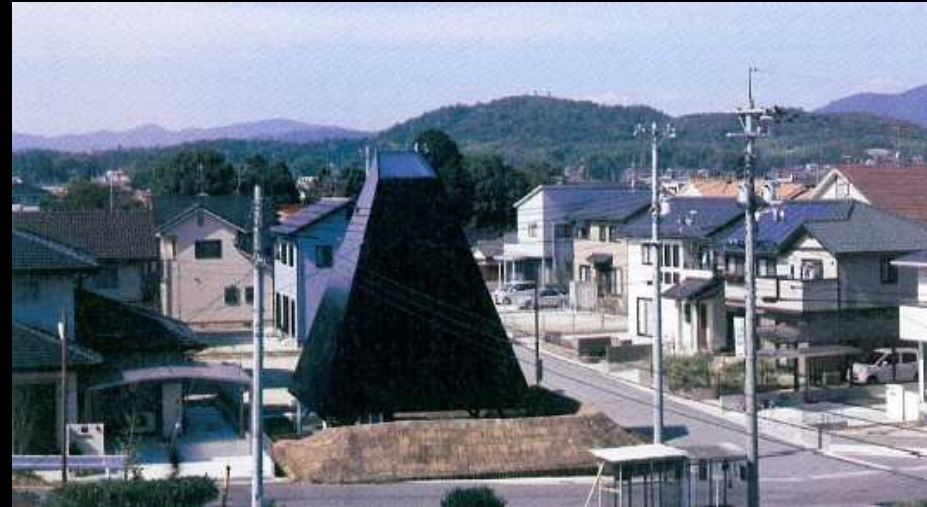
HOUSE, SAIJO, JAPAN ARCHITECT SUPPOSE DESIGN OFFICE
