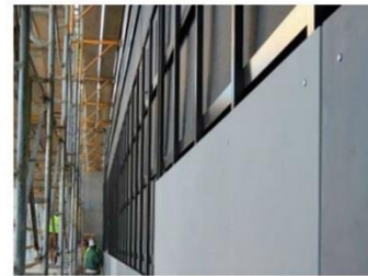
Rainscreen | Exposed Direct Fastener
