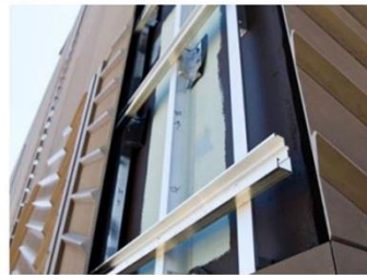
Rainscreen | Undercut Anchors
